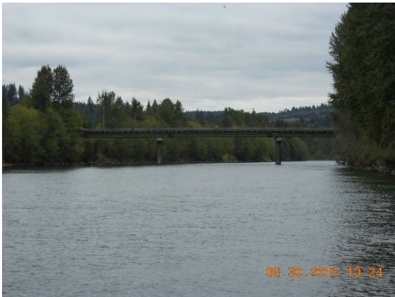
Photo 11 - Looking downstream at Hwy 411 bridge
