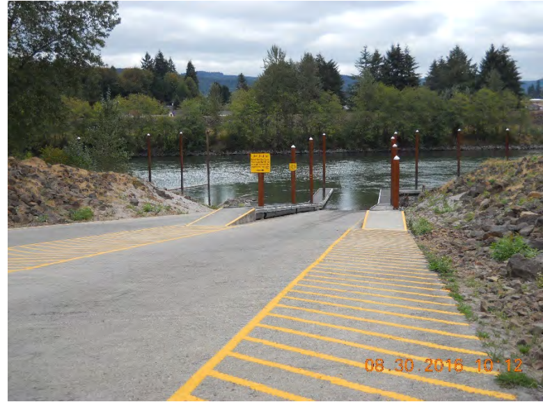
Photo 2 – View from top of ramp
