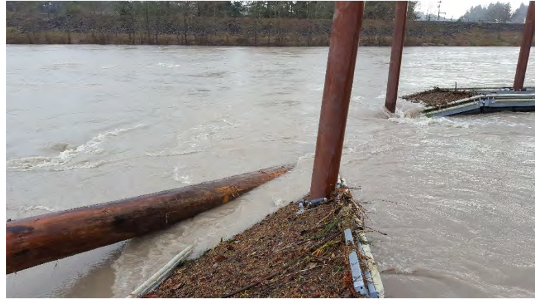
Photo 16 – Debris on floats during December 9, 2015 high water
