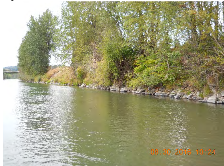
Photo 12 – riprap protection along downstream bank
