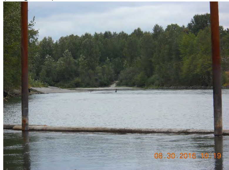
Photo 8 – Looking upstream from end of boarding floats
