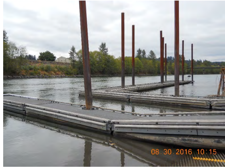
Photo 6 – Boarding floats (foreground) and transverse float (background)
