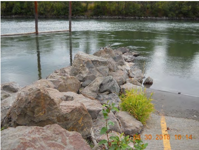
Photo 3 – Riprap protection added after Dec 2015 high water
