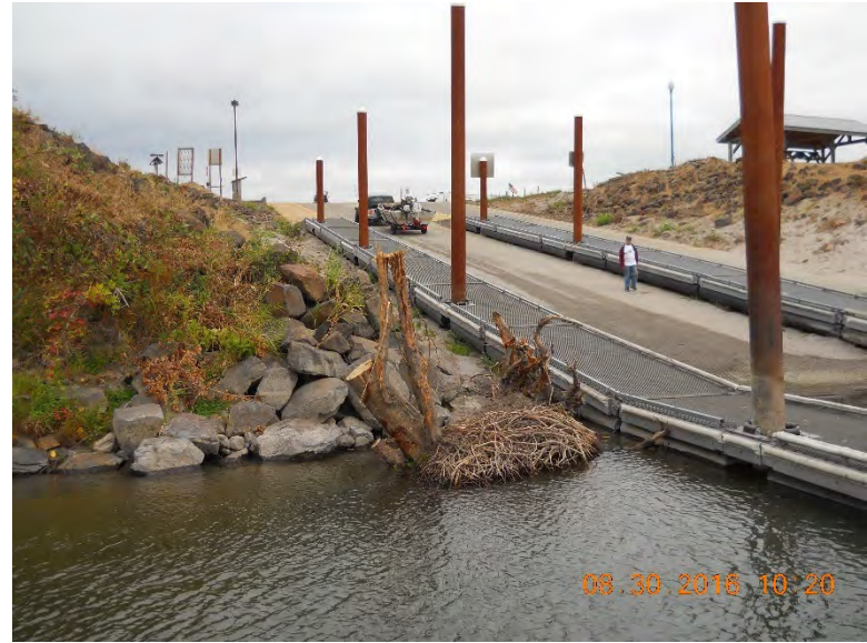
Photo 10 – looking at base of ramp and debris from Dec 2015 high water
