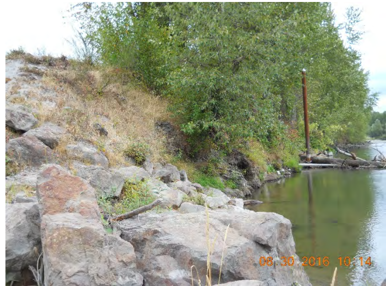
Photo 4 – Looking upstream along left bank
