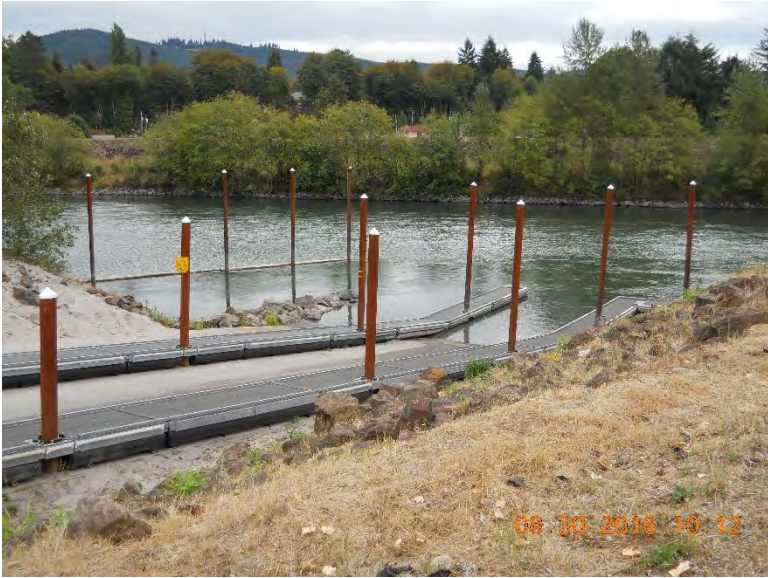
Photo 1 – View of boat ramp from parking area
