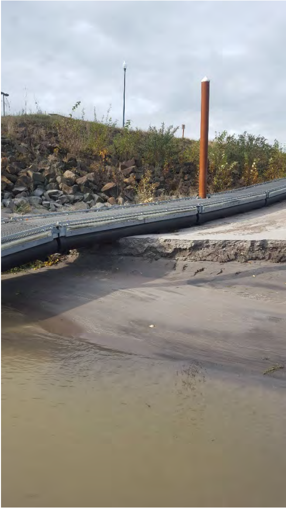
Photo 13 – Sediment deposits from December 9, 2015 high water
