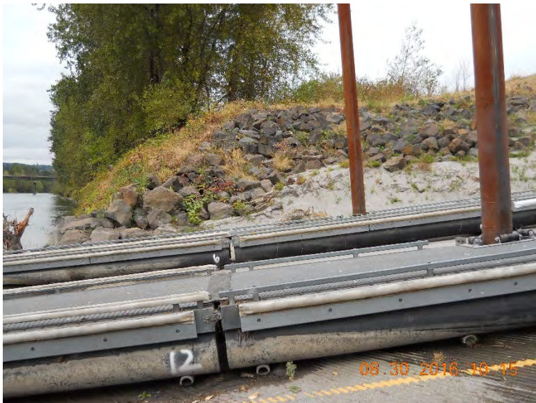
Photo 7 – Boarding floats and marks from sediment deposition
