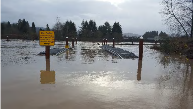
Photo 15 – December 9, 2015 high water
