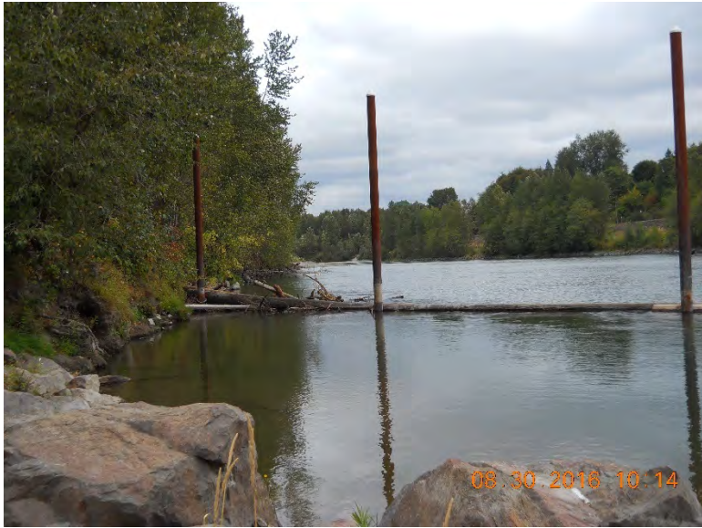
Photo 5 – Pile and log debris deflector
