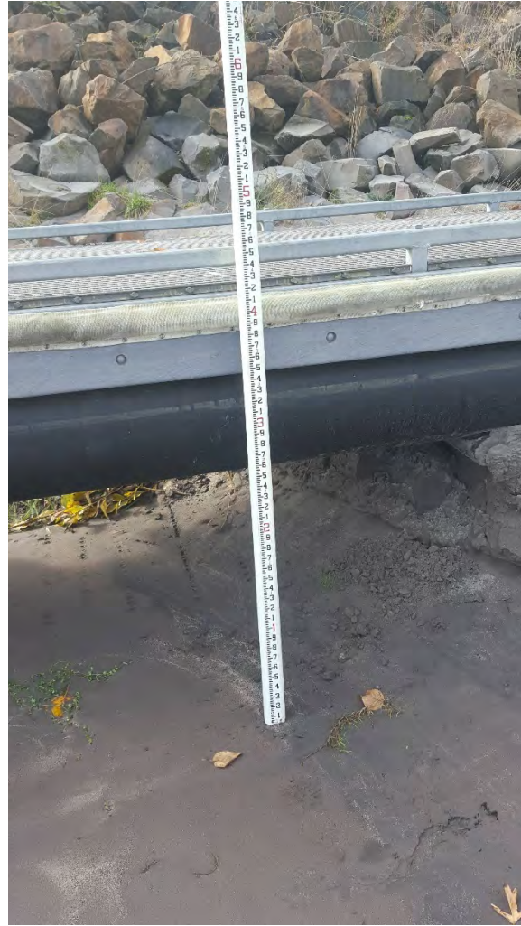
Photo 14 – Sediment deposits from December 9, 2015 high water
